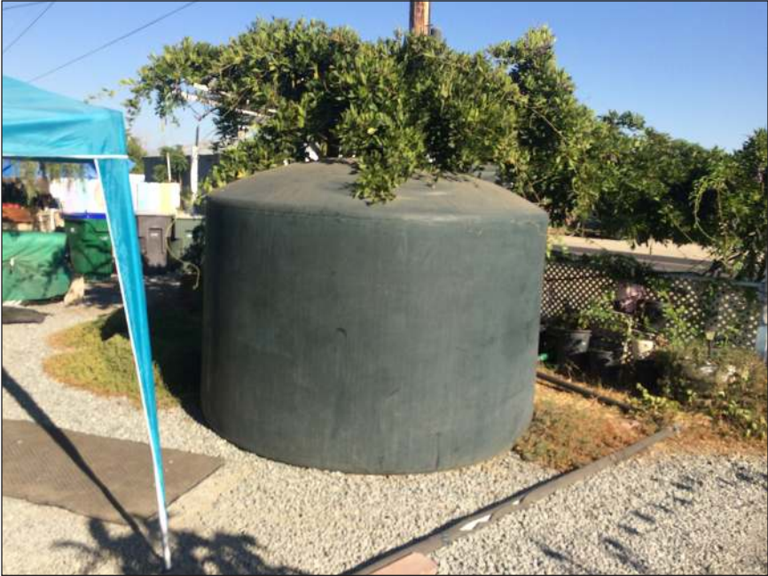
Figure 8.—Personal tank connected to household plumbing. Photo by author.
