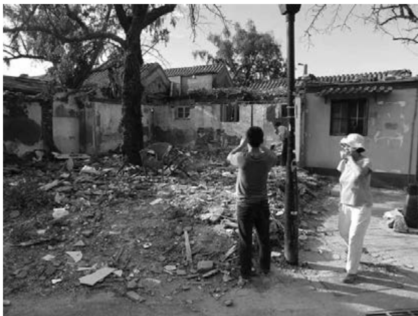
Figure 4.1 Demolition of dilapidated houses in front of the Drum Tower
