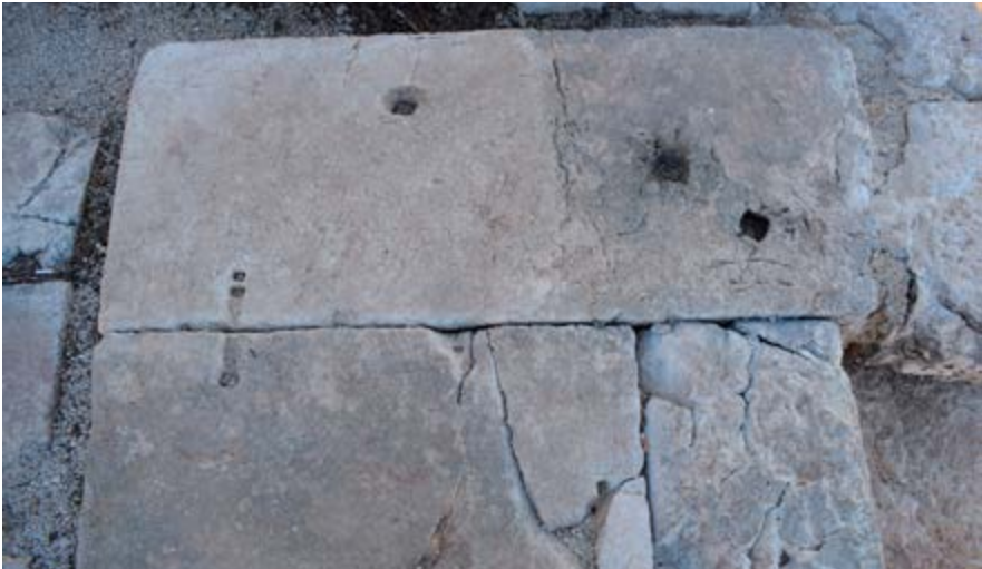
Fig. 2. The presence of clamp- and/or dowel-holes in slabs can help in identifying the original location of monuments.
